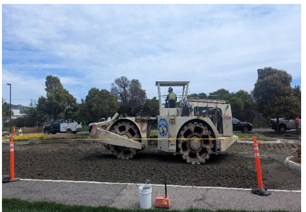
Photo 8: Cement base treatment equipment used for compaction.
