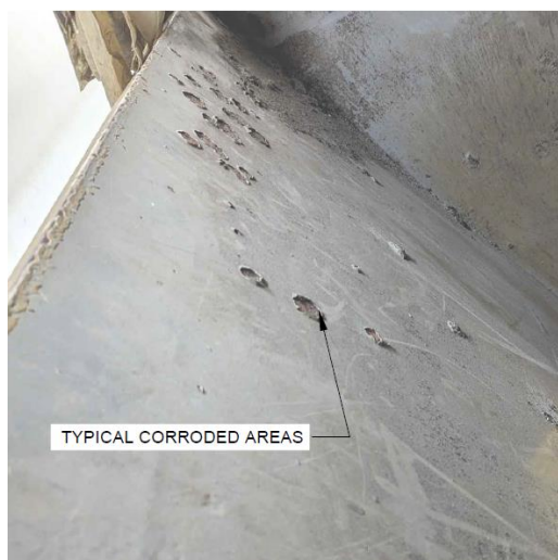
Figure 1: Corroded areas inside hopper
