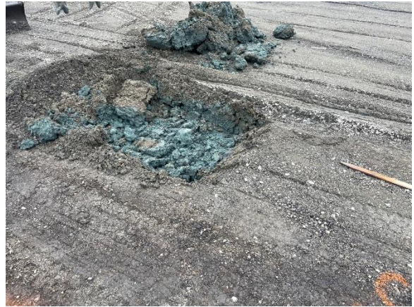
Photo 4: Unstable clay layer (young bay mud) beneath subgrade.
