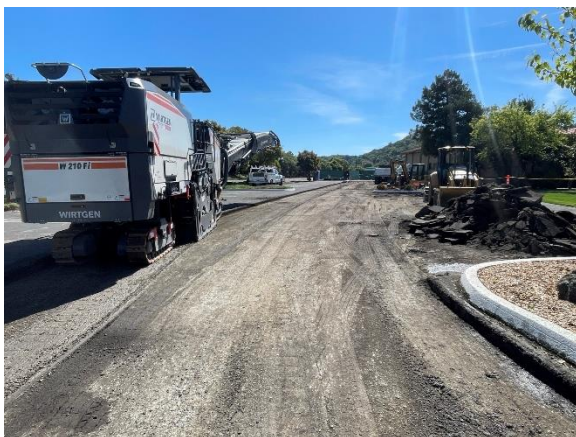
Photo 1: Grinding to remove asphalt surfaces.
