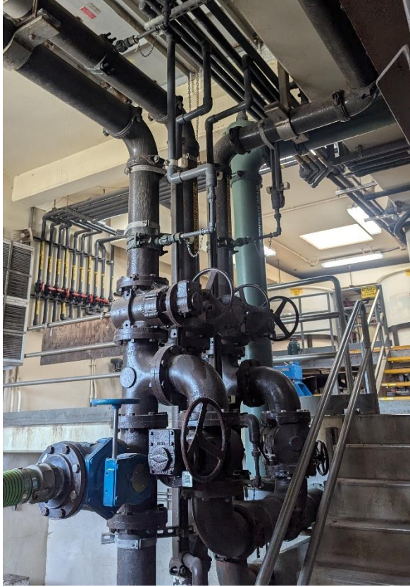
Figure 1: DeZurik plug valves and Victaulic fittings and couplings on the centrifuge feed and centrate piping
