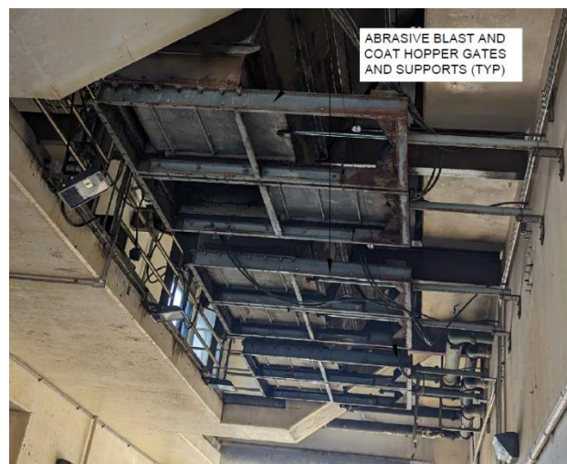
Figure 2: Corroded hopper gates
