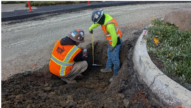
Photo 5: Potholing unmarked utilities.
