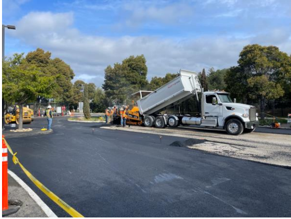
Photo 9: New pavement installation.
